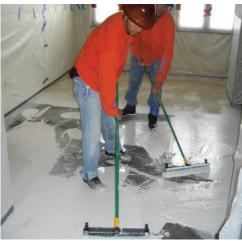
MAXXON® DPM (Damp Proof Membrane) is a unique 2-component, moisture tolerant, extremely high density, chemically enhanced epoxy-based product which prevents the passage of water vapor and moisture through concrete floors and walls on or below grade. DPM eliminates delamination of adhesives, floor coverings and coatings. DPM also prevents capillary infiltration of oil or other chemicals from the ground and can be used to treat oil-contaminated slabs.
