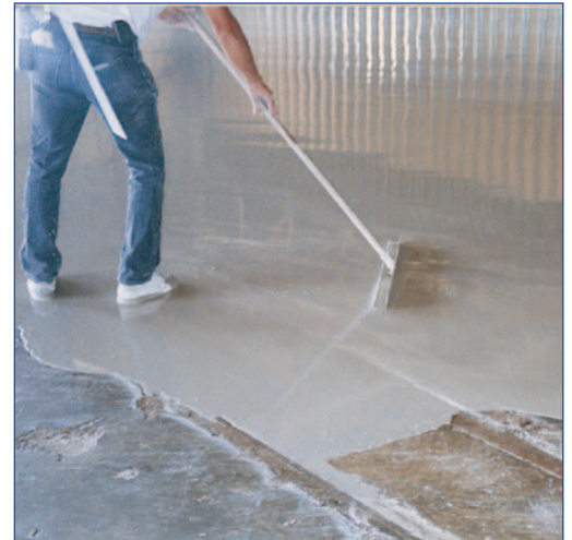
ON THE LEVEL — Level-Right/PLUS/FS-10 make old, rough, pitted concrete floors smooth and level.
