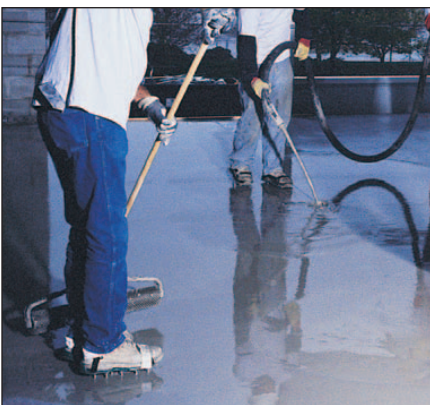
As Level-Right/PLUS/FS-10 level, they fill in worn, cracked and damaged areas completely.
