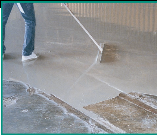
Level-Right makes this old, rough, pitted concrete floor smooth and level.
